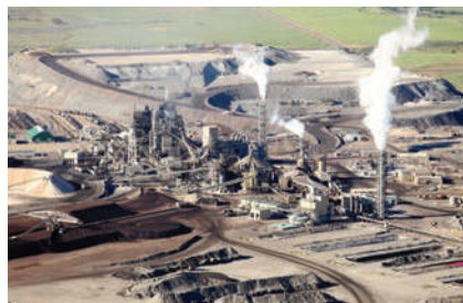
Mines and construction sites
